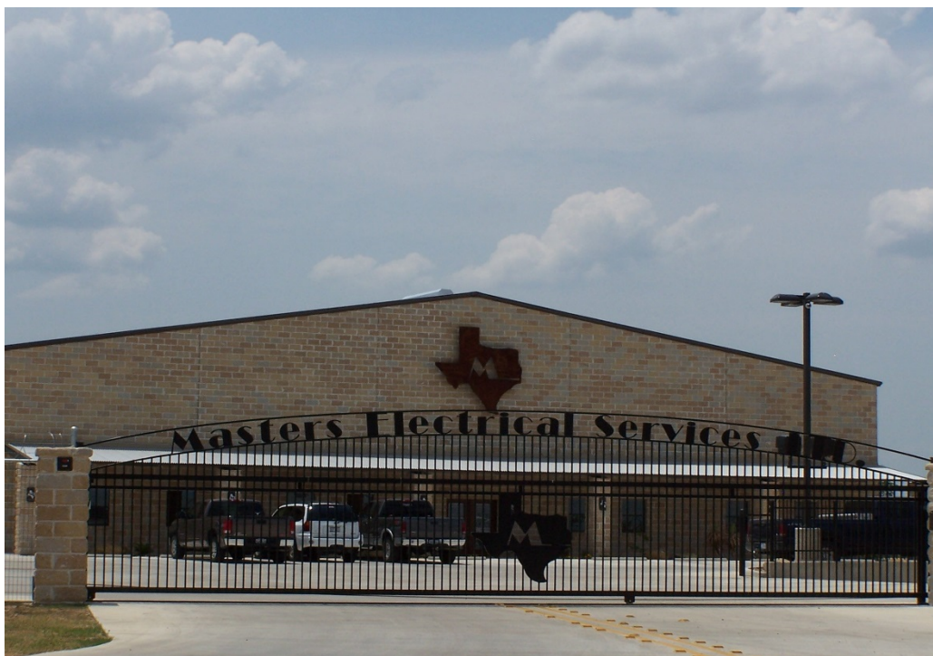
MASTERS ELECTRICAL SERVICES LTD. 4239 W. IH-10; SEGUIN, TEXAS 78155
